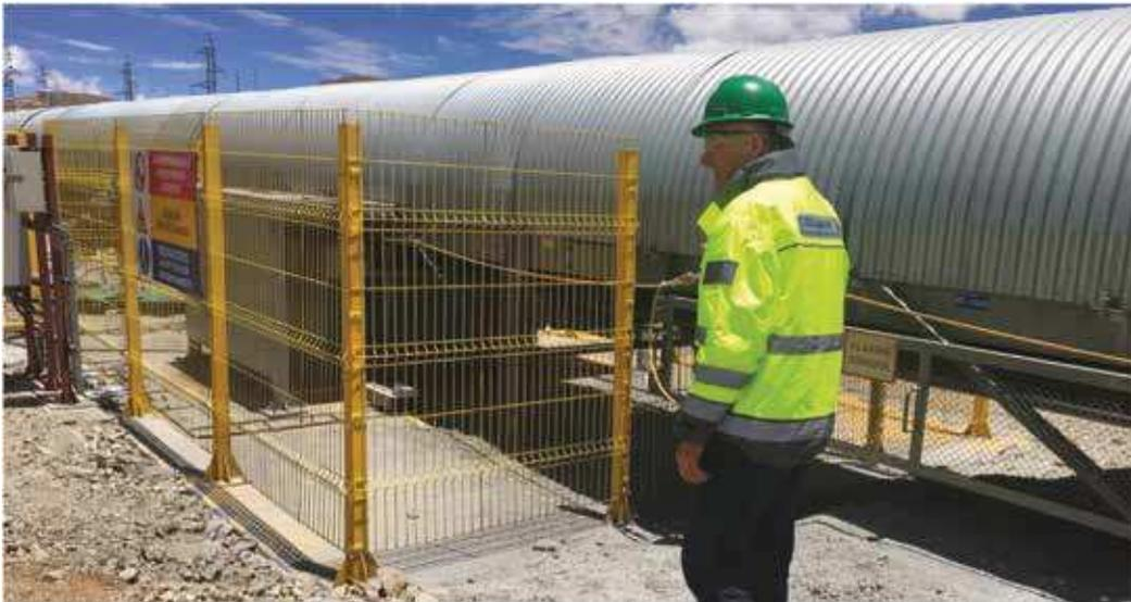
virtually every cubic millimeter of the belt is captured. That way, the X-ray system can be integrated into the IIoT. A reconciliation with the control units of other conveyor components is enabled. The optimal time of the next maintenance stop can be scheduled.
